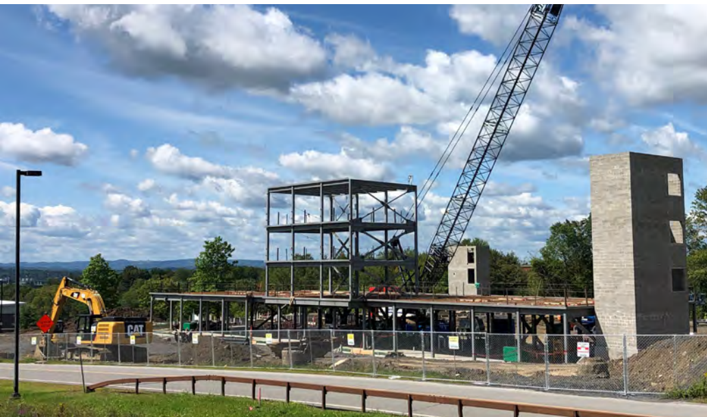
Construction begins on SUNY Poly’s Hilltop Residence Hall
